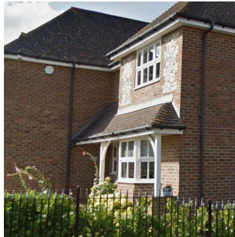
Figure 71: Bay window under a pitched porch.
