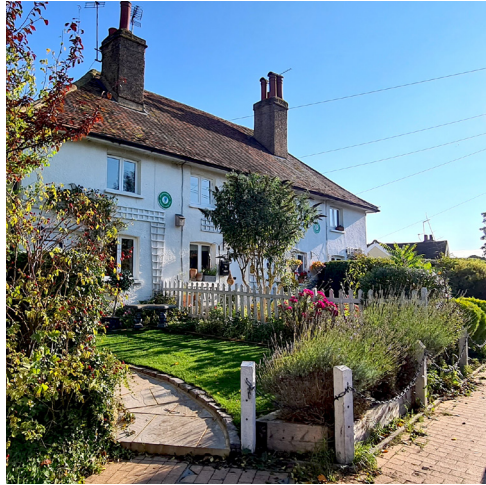
Figure 39: Planters acting as a boundary treatment.
