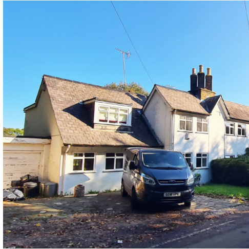
Figure 74: Double-storey side extension.
