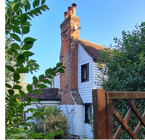
Figure 62: Brick chimney connected to the ground.
