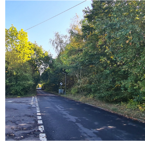
Figure 4: View along Wood Street, leading under the M25.
