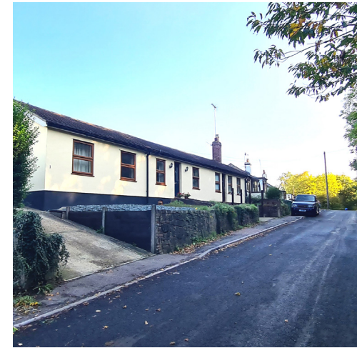
Figure 30: Bungalows with access from the street and a view to the Green Belt from the back gardens.
