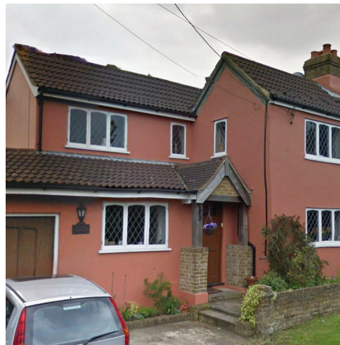
Figure 78: Double-storey side extension.
