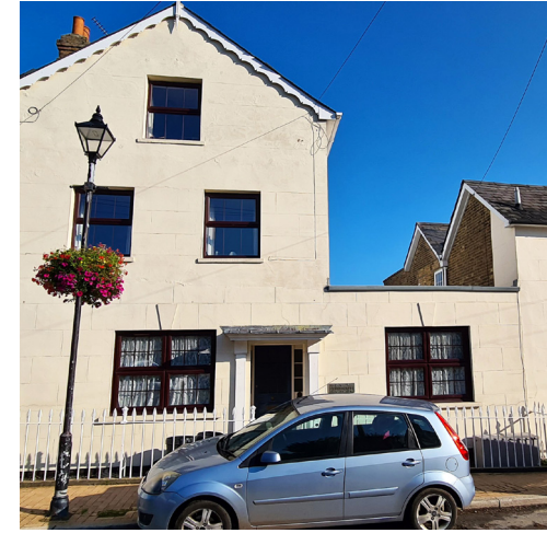
Figure 27: Building fronting onto the road.
