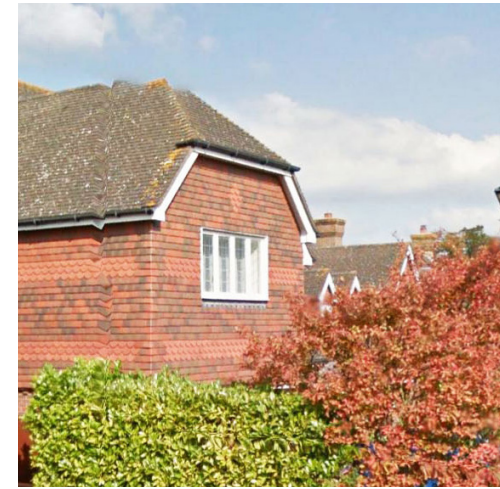
Figure 86: Vertical hung tiles used on facade of the building.
