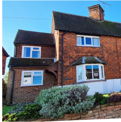
Figure 75: Double-storey side extension.
