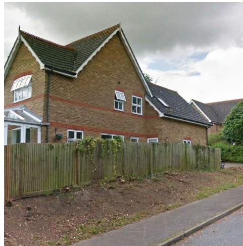
Figure 29: High fence fronting onto the road, this should be avoided.
