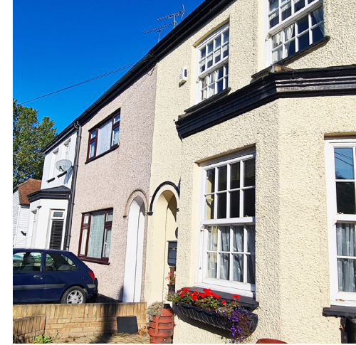
Figure 69: Windows evenly spaced out and in line with each other.
