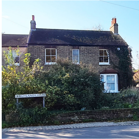
Figure 60: Pitched roof with symmetrical chimneys.
