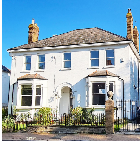
Figure 68: Symmetrical bay windows.
