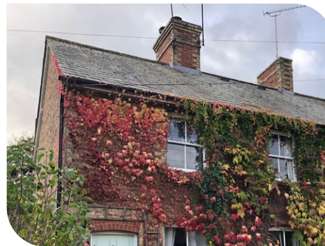
Welsh slate roofs
