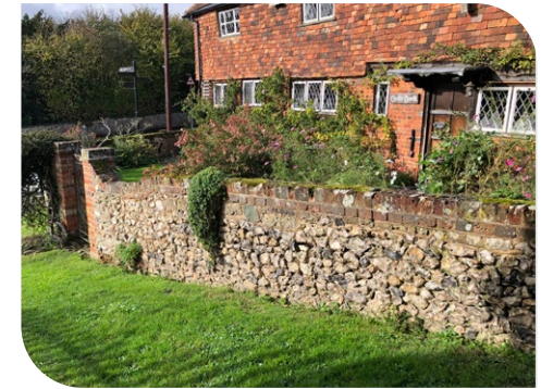
Knapped flint walls
