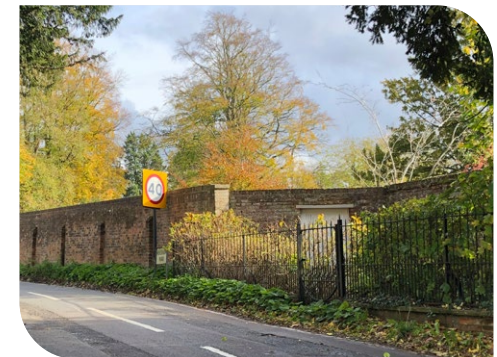
High brick walls
