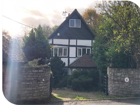
Timber framed buildings
