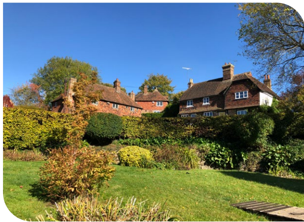
Townscape views within the Conservation Area illustrate the mix of building types, forms and materials and give a sense of the spatial character and architectural quality of the village. Trees and other greenery play an important part in these views.
