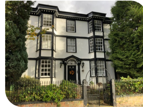
Structural use of timber and painted lime render
