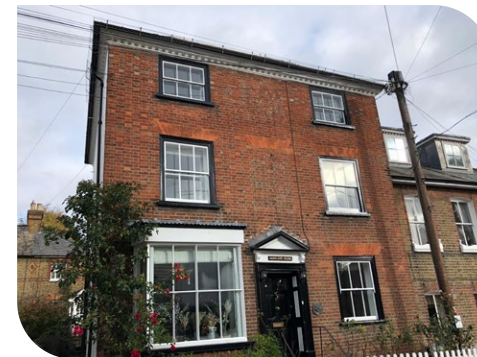
Sash windows and panelled timber door
