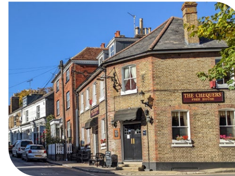
Welsh slate roofs
