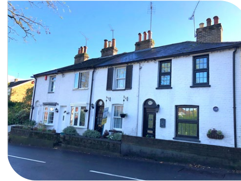
Welsh slate roofs
