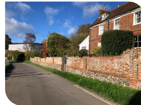
Flemish bond brickwork
